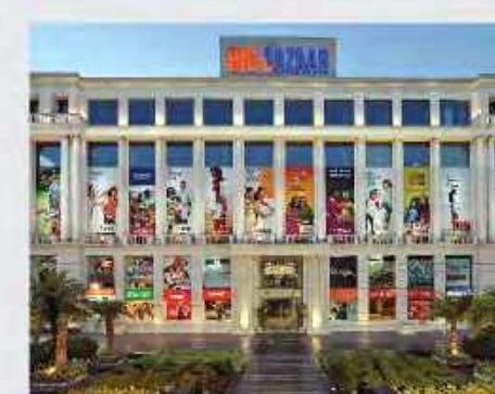
SHALIMAR ELLDEE PLAZA BHOOTNATH MARKET, LUCKNOW
