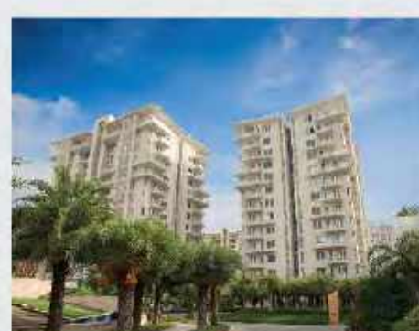
SHALIMAR GALLANT MAHANAGAR, LUCKNOW UPRERAPRJ3168
