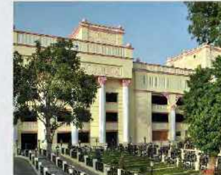
MULTILEVEL PARKING HAZRATGANJ, LUCKNOW
