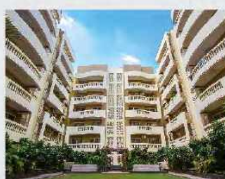
SHALIMAR DWELLING AP SEN ROAD, LUCKNOW
